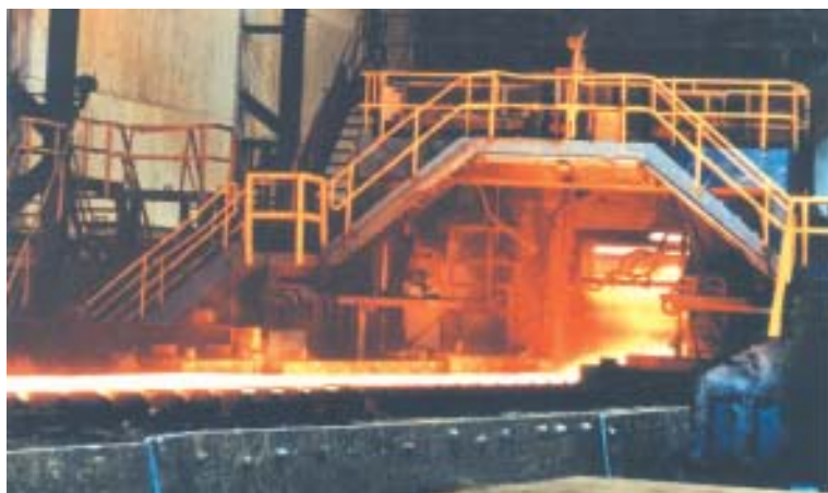
Stands R2 and R3 of the roughing mill at Corus Llanwern's hot strip mill were restored to original tolerances using in-situ machining expertise by Metallock
