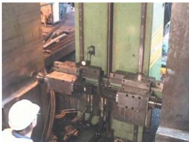
The main machining emphasis was to restore vertical wear plate faces and modify mill housing windows on Stand H4 to permit the fitting of 'E' blocks. Picture shows extending window width, both sides simultaneously, for this modification.
